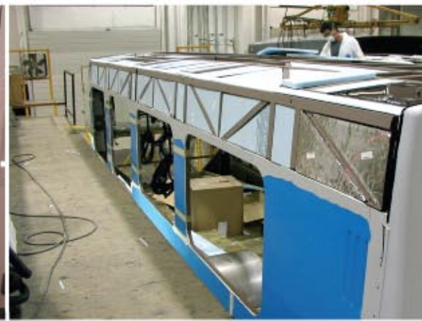
Bus shell assembly using a combination of Bostik polyurethane and SMP products
